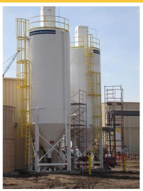
Westpro designs and manufactures turnkey modular Reagent Preparation & Dosing systems. These systems can be configured to handle both bulk chemicals and liquid reagents, and deliver them to the process at the desired solution strength.
